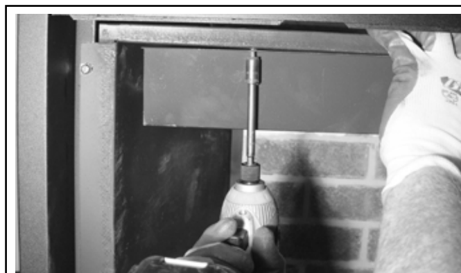
Figure 1 - Remove the lintel (specified models only)
