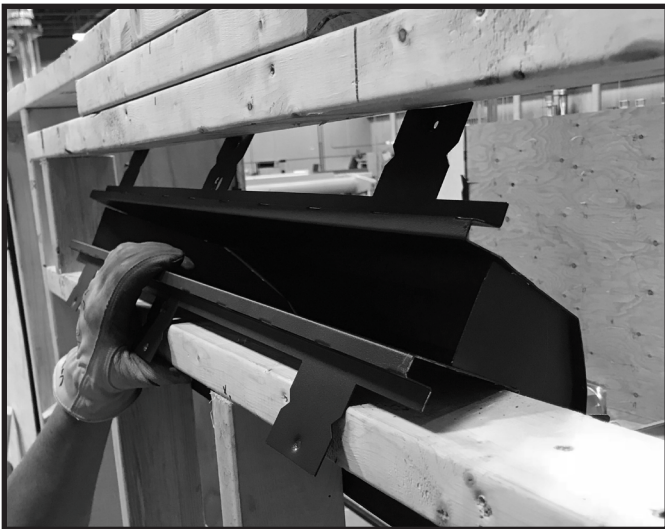
Figure 5.17 Place Plenum From Inside of the Chase
