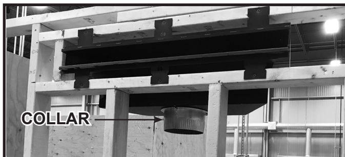
Figure 5.25 Install Collar(s) to Bottom of Plenum
