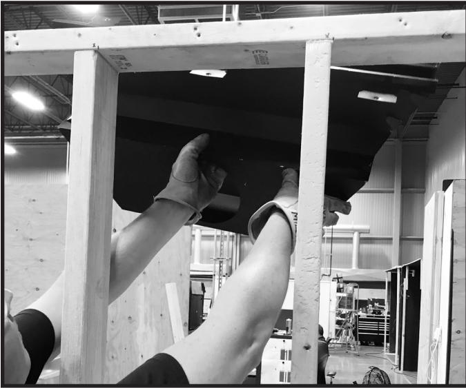
Figure 5.16 Rotate Plenum to Horizontal Orientation
