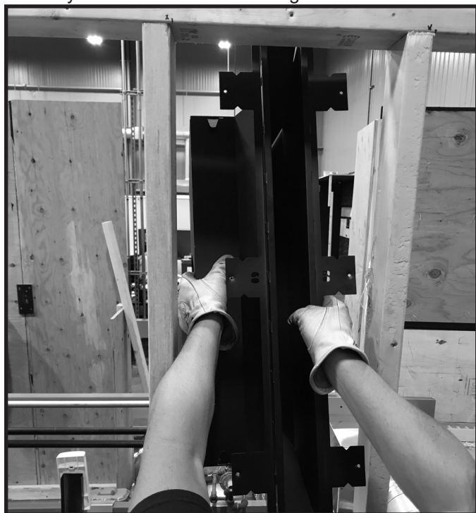
Figure 5.15 Turn Plenum Vertically to Clear Framing Studs
