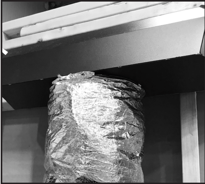
Figure 5.26 Install Flex Venting to Collar on Bottom of Plenums
