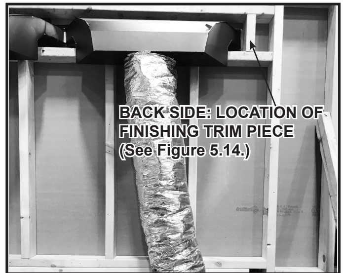
Figure 5.29 Flex Vent Installed with No Kinks
