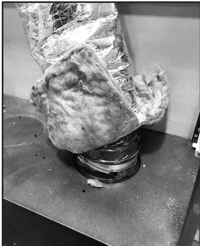
Figure 5.27 Install Flex Venting to Appliance
