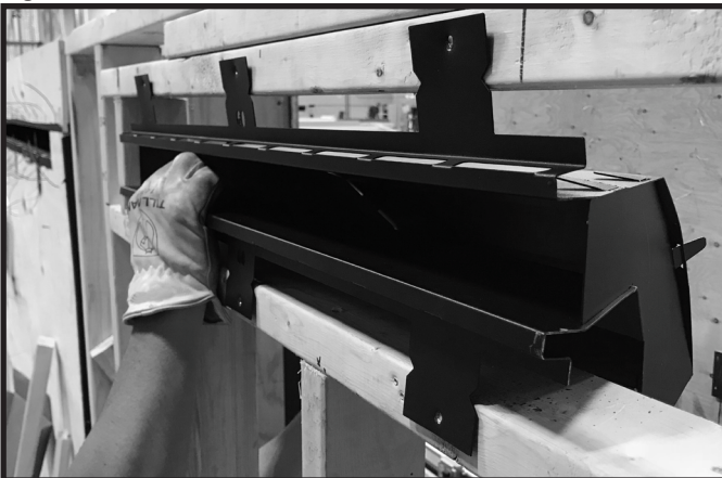
Figure 5.18 Position Plenum
