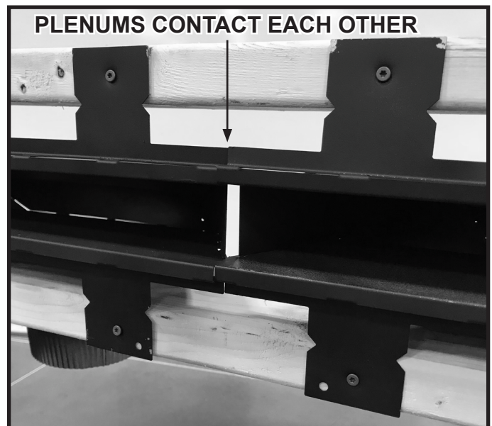
Figure 5.21 Plenums Contact Each Other
