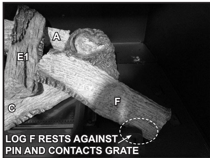
Figure 10. Log F Installed
