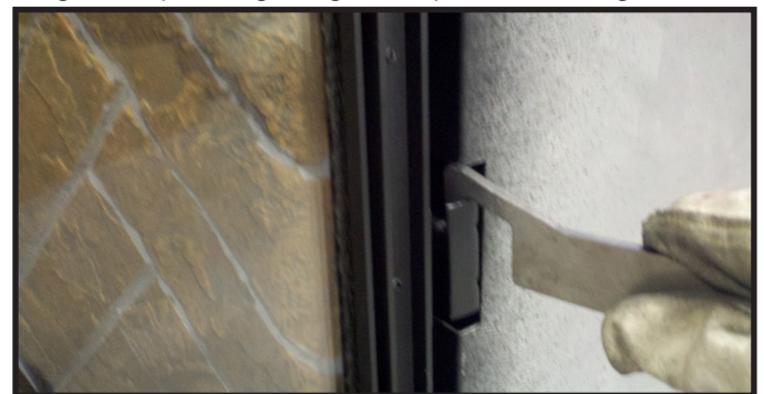
Figure 11.7. Securing Side Glass Clips
