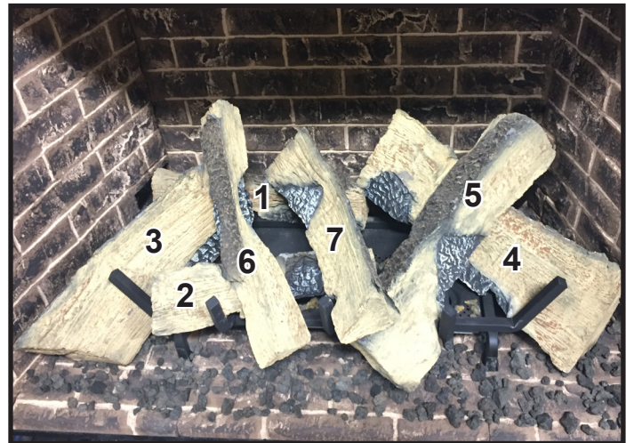
Figure 16. Log Set Installed
