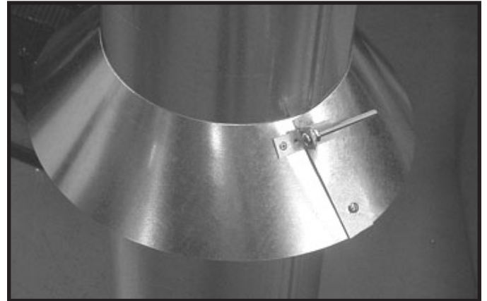
Figure 7.12 Insert Bolt into Brackets
