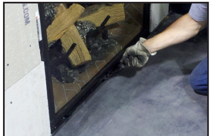
Figure 11.8. Securing Bottom Glass Clips
