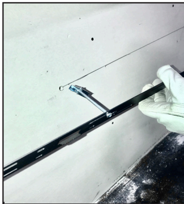
Figure 4.4 Toggle Bolt Installation through Mounting Bracket
