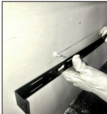
Figure 4.5 Installing Anchors in Hollow Wall
