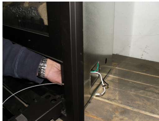
Figure 6 Installing the PPO Box (from outside of fireplace).
